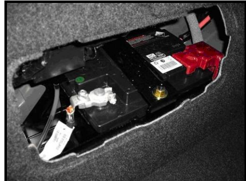
Interior trim removed
