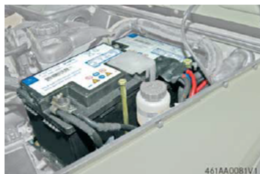
Figure 2: Vehicle Start Batteries, located beneath the vehicle bonnet
