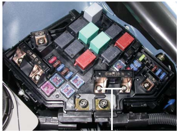
Main Fuse Assembly Screws
