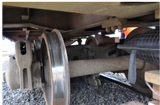
Carriage is lifted clear of the bogie, exposing the king pin.
