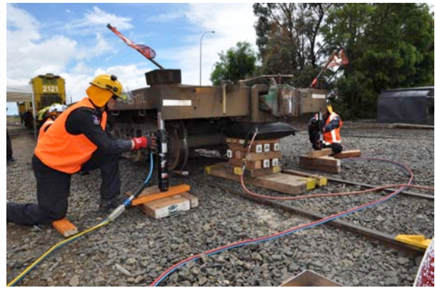
Carriage lift, the airbags provide most of the lift, the power rams help keep the wagon level during the lift.
