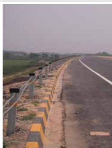
Gorakhpur Bypass Project NH-28 – 5 KM Client: Gammon India Ltd
