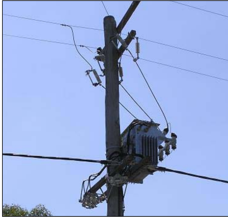
Figure 15 SWER pole substation
