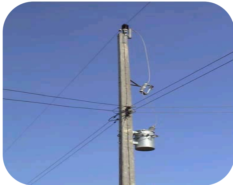
Figure 15 SWER pole substation
