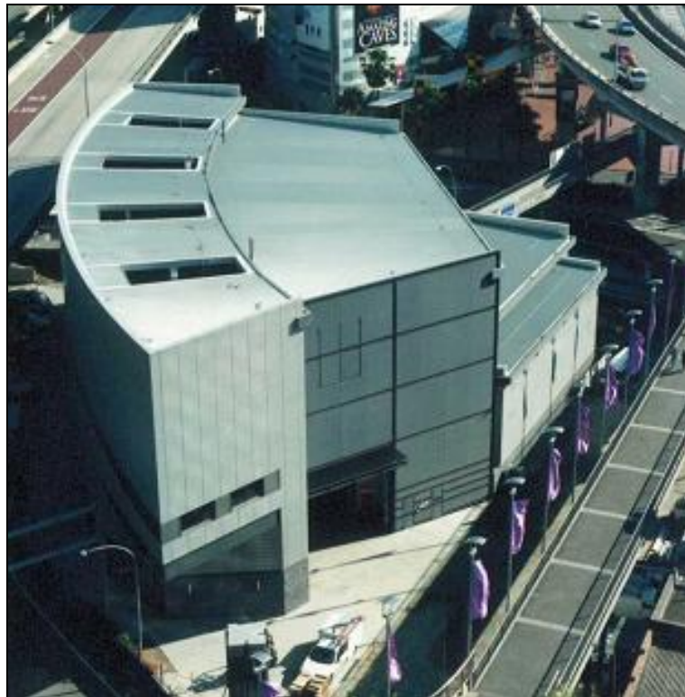
Figure 8 Enclosed zone substation example—City Central
