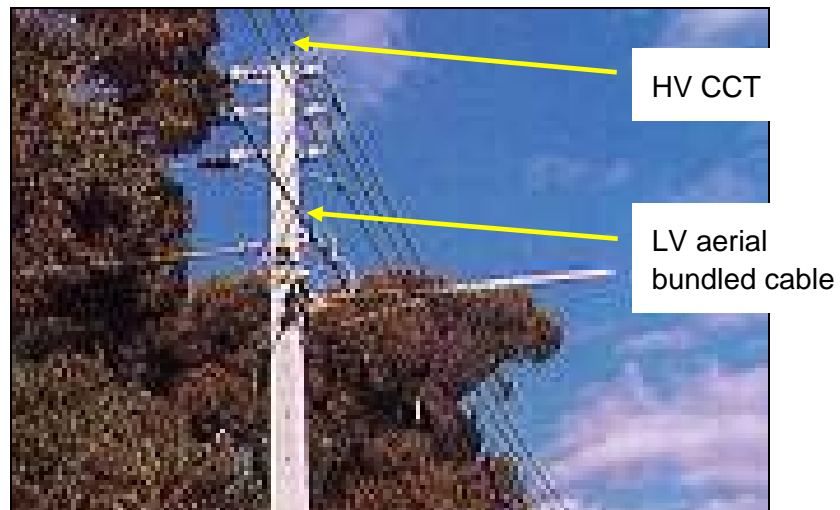
Figure 22 Low voltage aerial bundled cable
